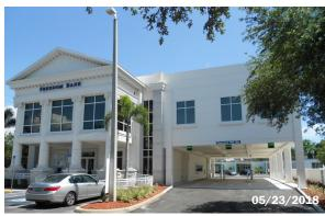
SCOPE OF WORK: Second story addition on steel columns over an existing drive-thru adding 3,168SF of office space. Renovations include enclosing existing second floor open air balcony to add more offices and admin space as well as renovations to reconfigure data, copy, conference & break rooms.
